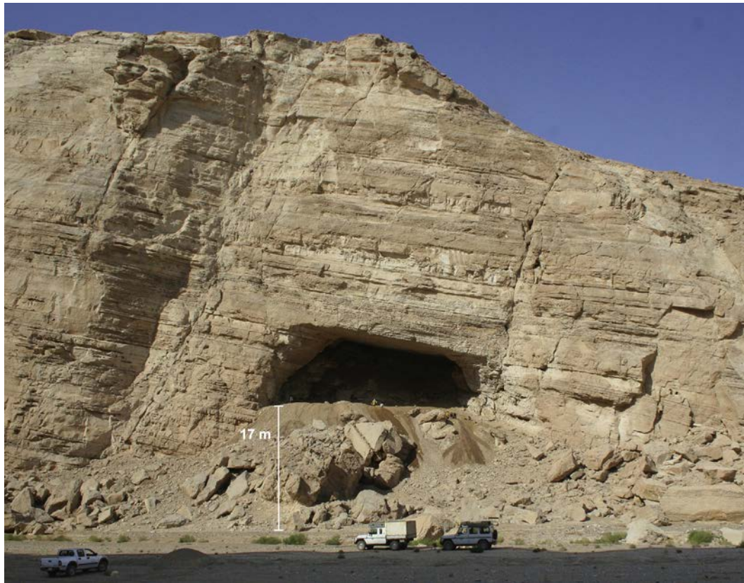
Fig. 2. Wadi Sodmein with the cave during the excavation in 2010; the present wadi floor is located around 17 m below the cave entrance.
